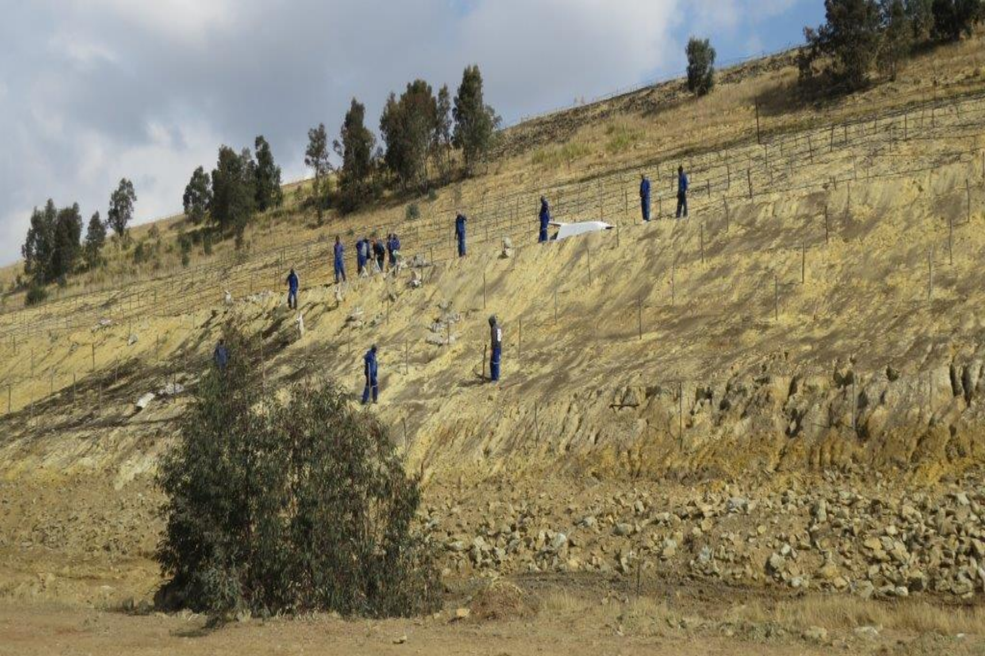
Workers from the local community preparing the slide slopes of the Crown TSF for grassing
