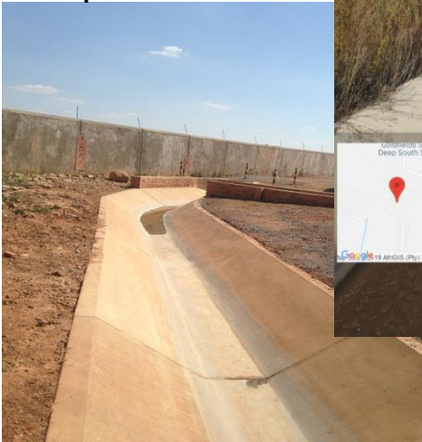
Concrete lined trench transition to buried pipe
